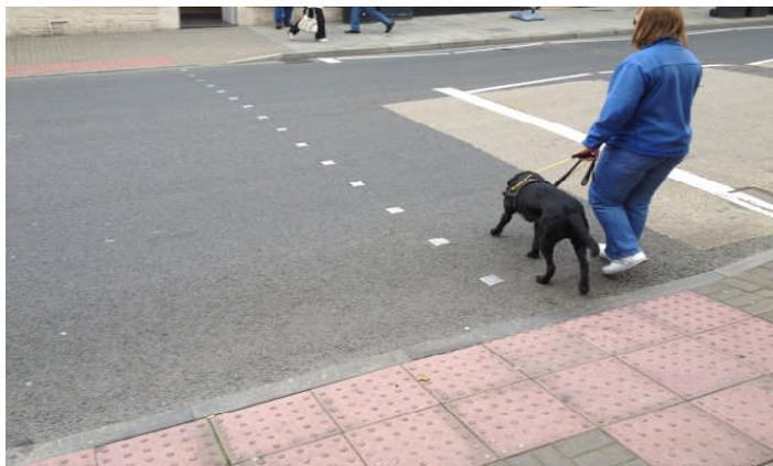
Depending on the position of the “push button box” the GDO may not be able to take up a central position again and will be forced to cross from the extremity of the paving. In the case of a cone being at distance from the crossing the guide dog owner
